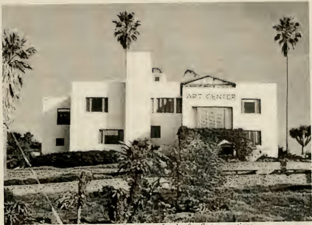
Fig. 3.2 – The Art Center, rear façade after first renovations.
